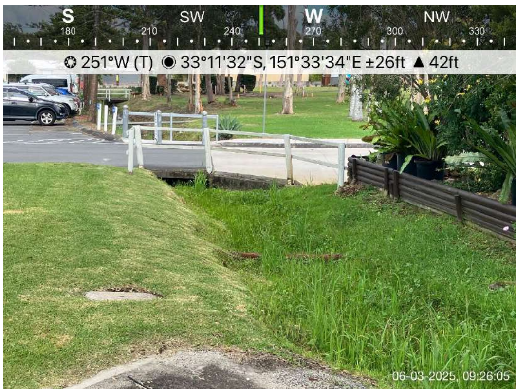
Photo Point 5 view of the offsite man-made drainage channel to the west that intersects the manufactured home estate and flows further west. The hydroline mapping does not follow this alignment, despite it being the only flow path to the south through the manufactured home estate.
