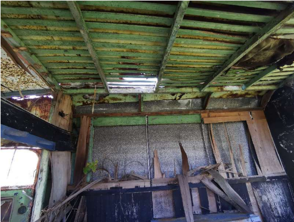
Photo 4.15 Inside of an old lorry which contains some potential shelter sites for fauna species
